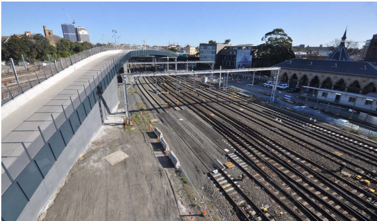
Figure 4: Completed Sydney Yard Access Bridge
