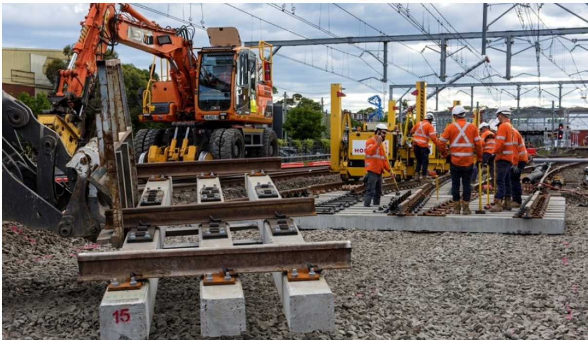
Figure 9: Track-laying as part of Sydenham Station Junction
