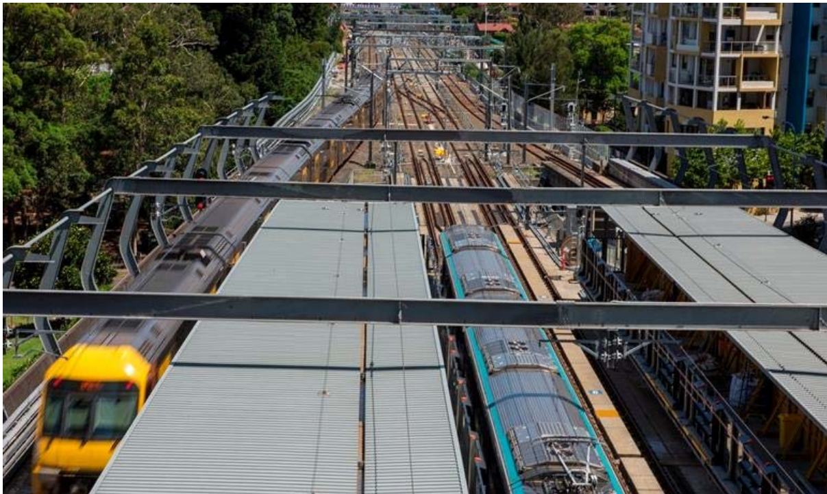
Figure 5: Sydney Metro and Sydney Trains Rolling Stock at Chatswood Station
