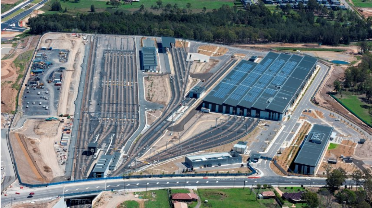
Figure 10: The Sydney Metro Trains Facility at Rouse Hill
