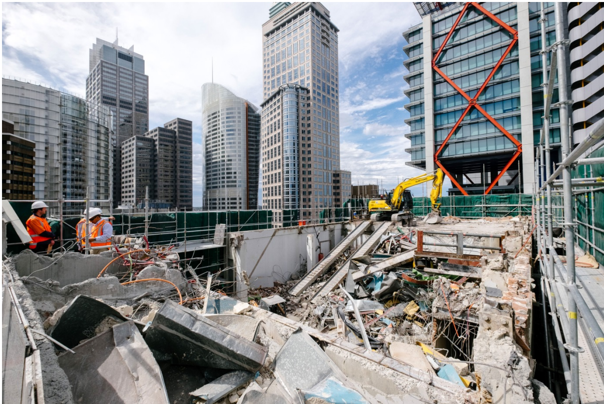
Figure 10: Structural Demolition at the Martin Place Station Site
