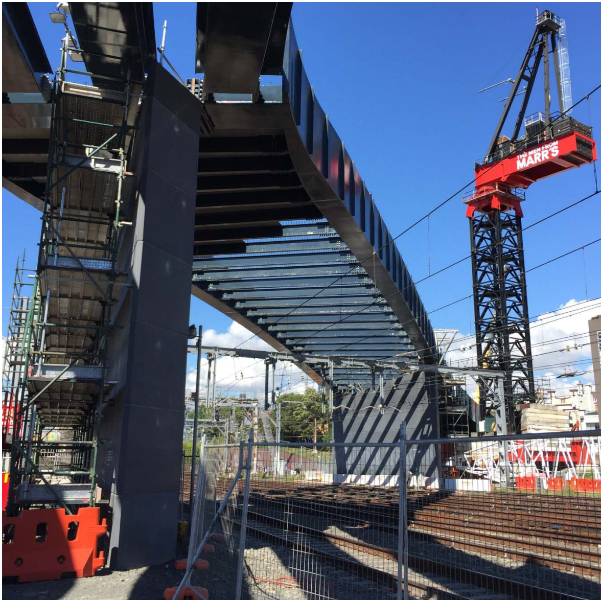
Figure 11: Construction of the Sydney Yard Access Bridge
