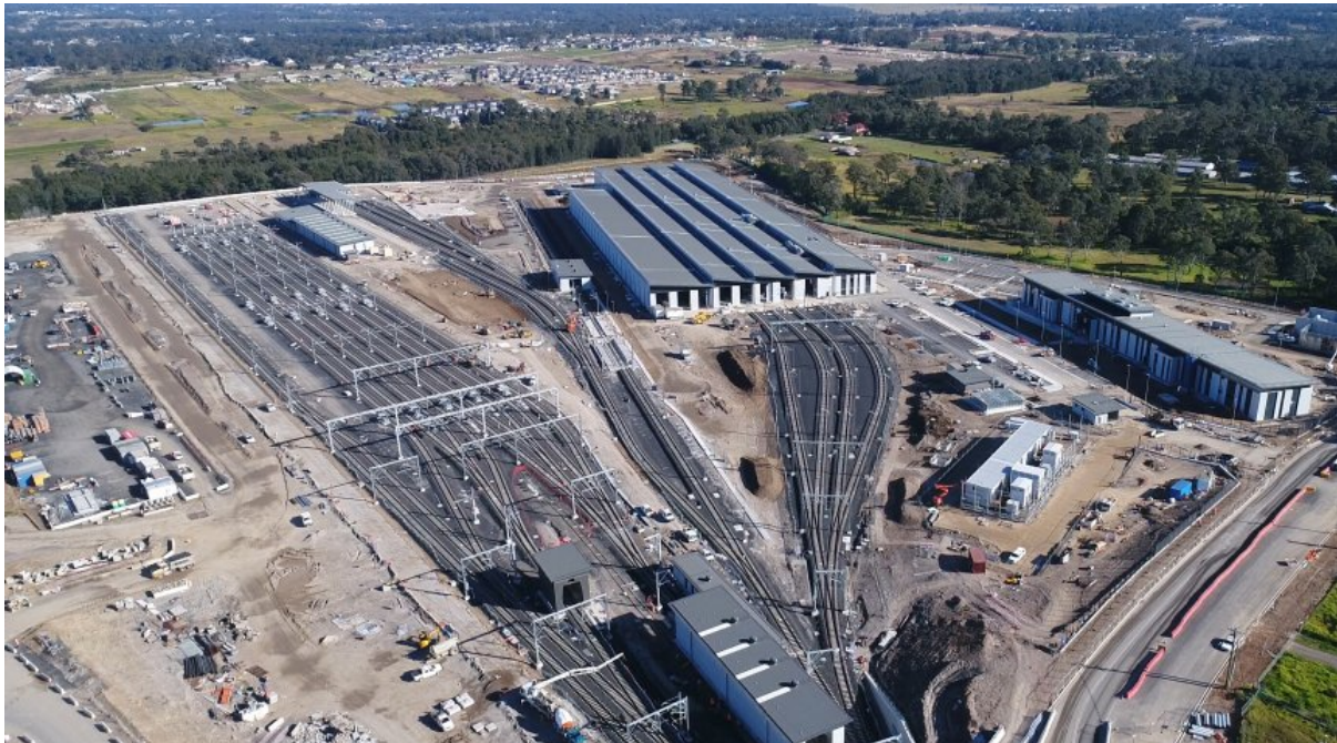
Figure 14: The Sydney Metro Trains Facility at Rouse Hill
