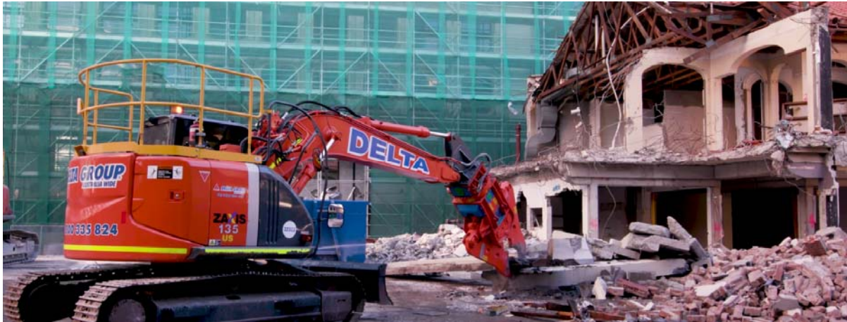
Figure 8: Structural Demolition at Tower Square (Victoria Cross Station Site)
