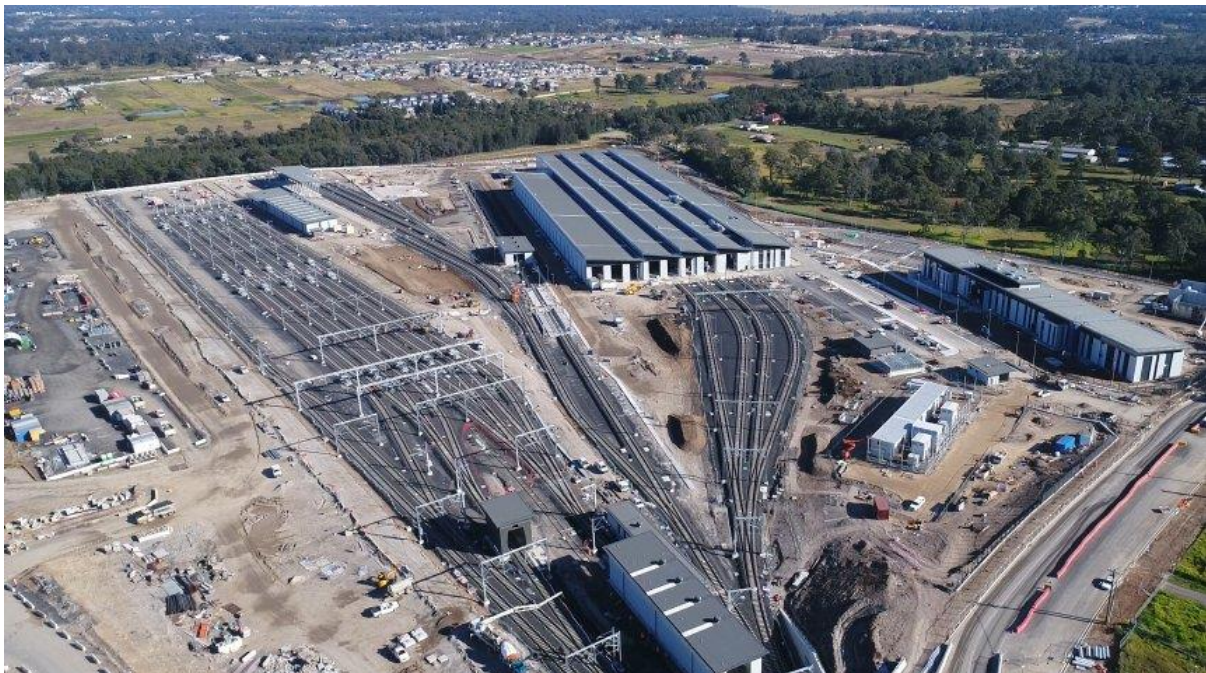
Figure 10: The Sydney Metro Trains Facility at Rouse Hill in July 2017
