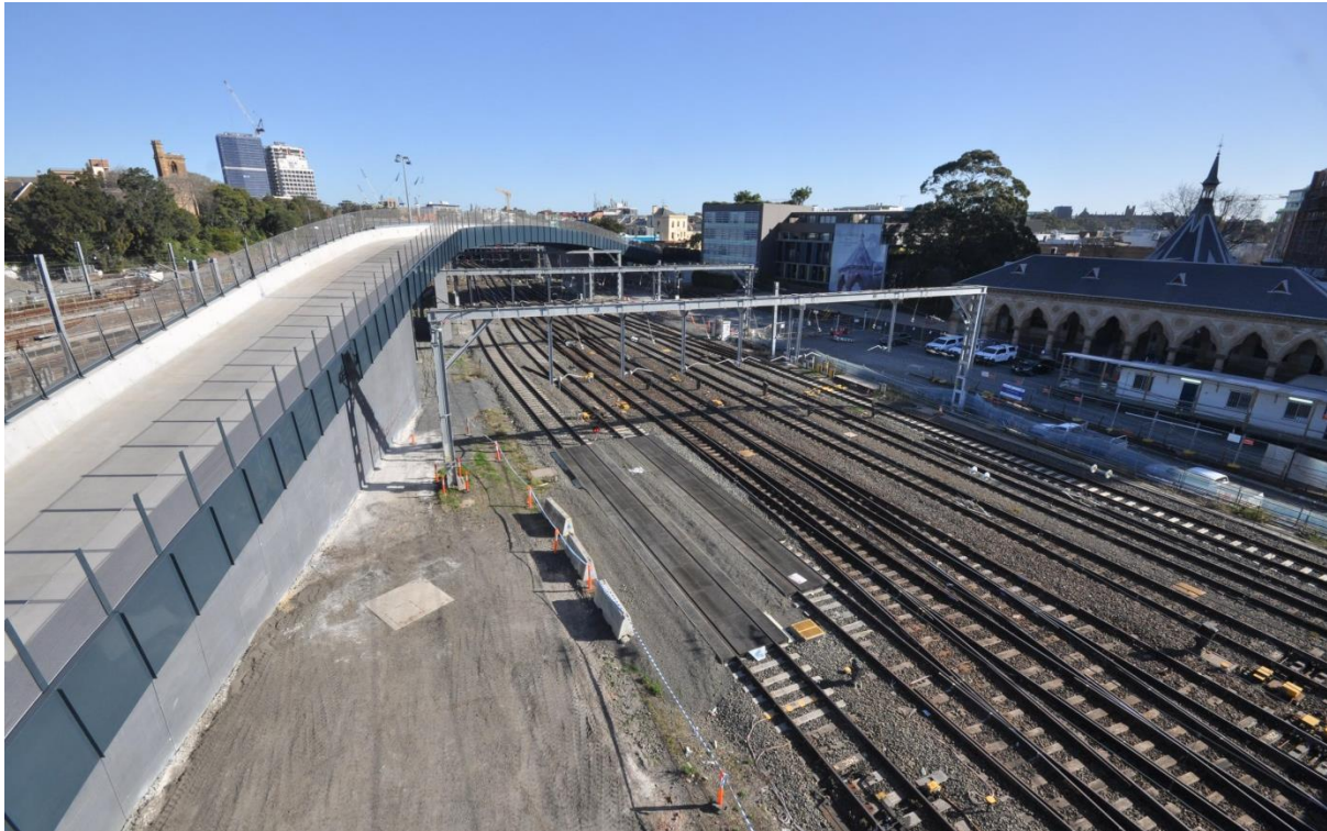
Figure 5: Completed Sydney Yard Access Bridge
