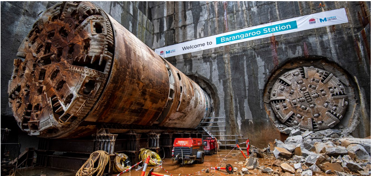
TBM Mum Shirl (right) breaks through at Barangaroo Station joining TBM Nancy inside the station box.
