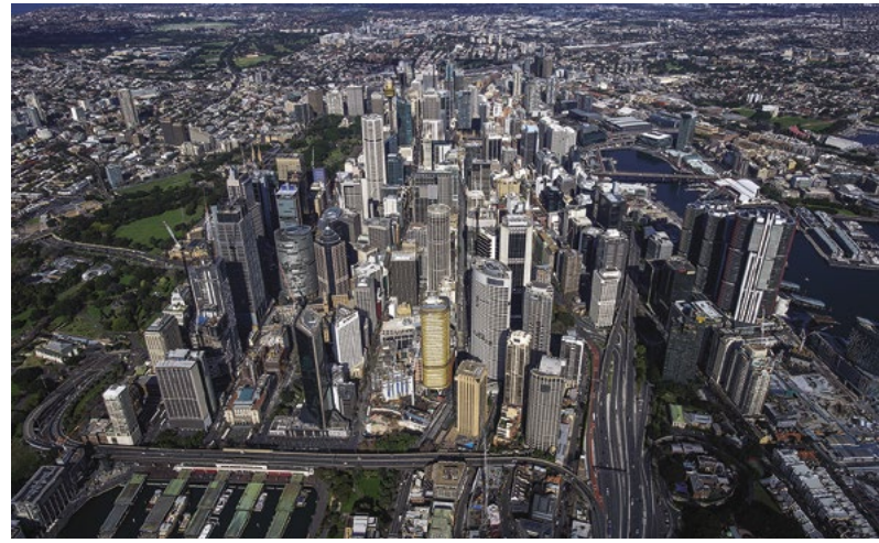
Aerial view of Sydney CBD.
