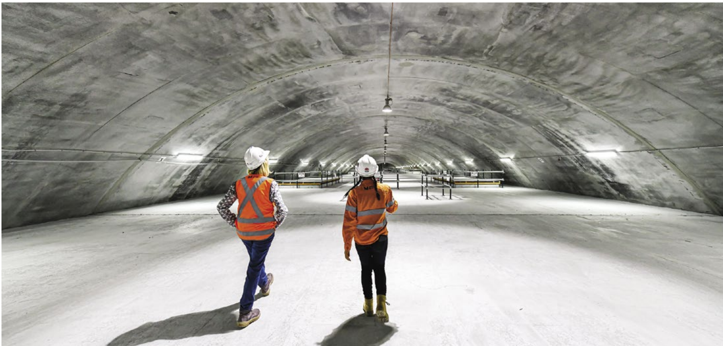
Cavern on the Sydney Metro City & Southwest project.
