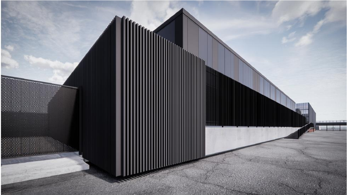
Figure 5 – View of Service Building (Hassell)
