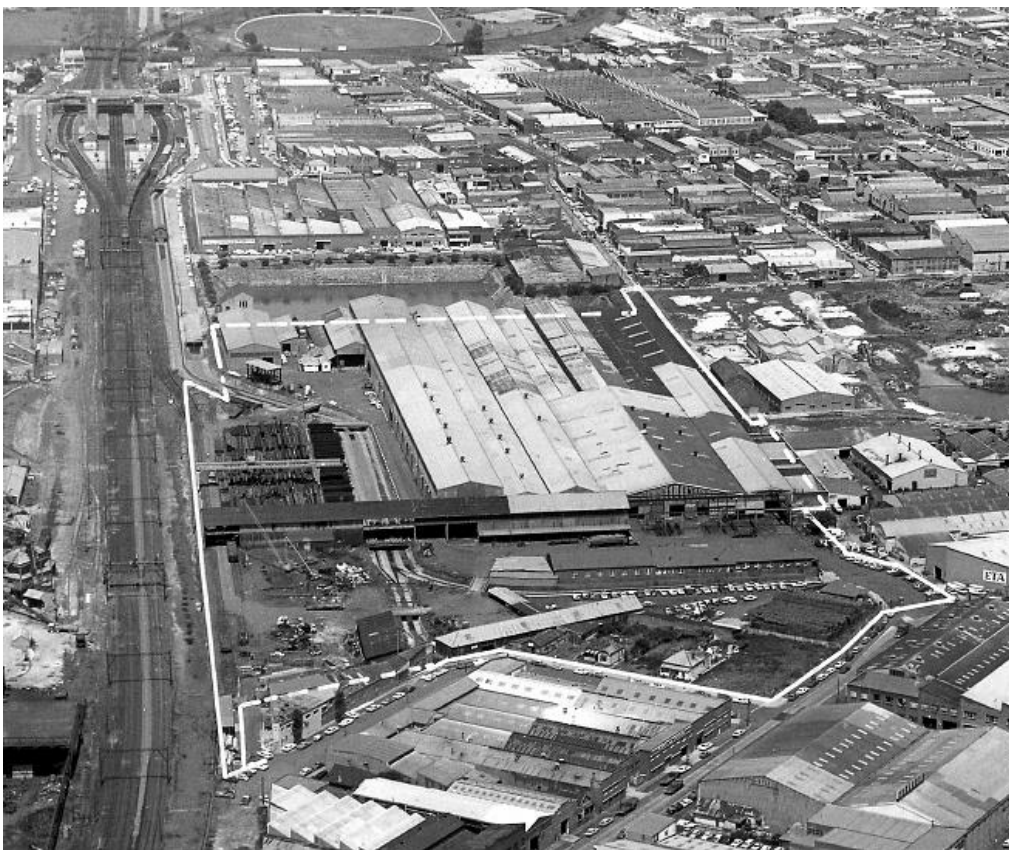
Figure 18 - The Sydney Steel Company site circa 1962.
