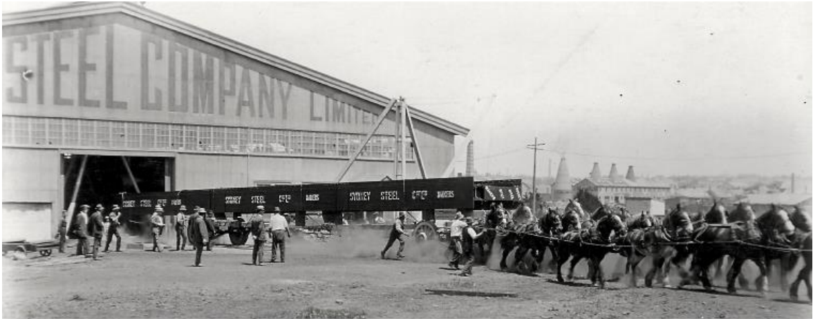
Figure 19 - The 44-ton girder fabricated for G & C Hoskins was 86-ft (26.2m) long, 8-ft (2.4m) deep and 3-ft (0.9m) wide. A custom-made limber drawn by 45 hand-picked horses was used to transport it to a rail siding near Sydenham Station in April 1919.
