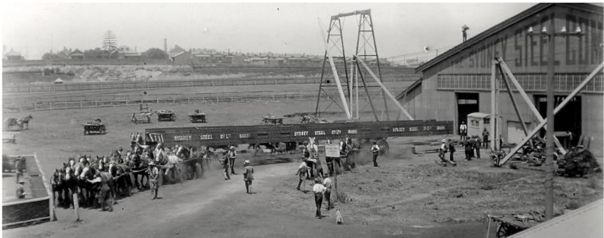
Figure 20 - The 44-ton girder fabricated for G & C Hoskins was 86-ft (26.2m) long, 8-ft (2.4m) deep and 3-ft (0.9m) wide. A custom-made limber drawn by 45 hand-picked horses was used to transport it to a rail siding near Sydenham Station in April 1919.
