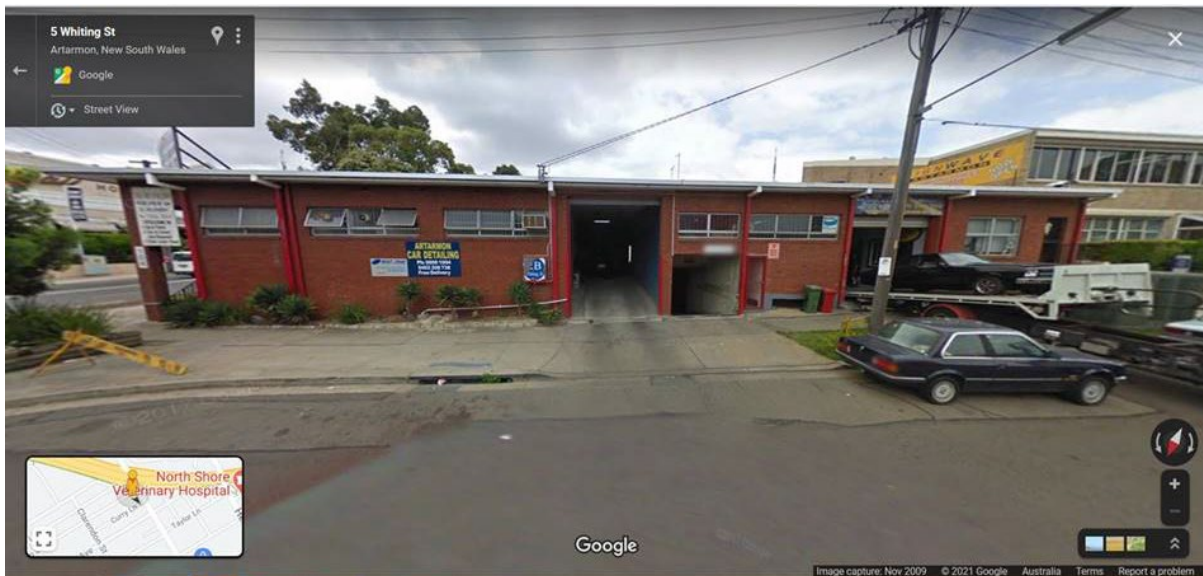
Figure 4-9 Site Contextual Photo from Whiting Street – Google Maps view from November 2009 (prior to demolition of existing building on the site)
