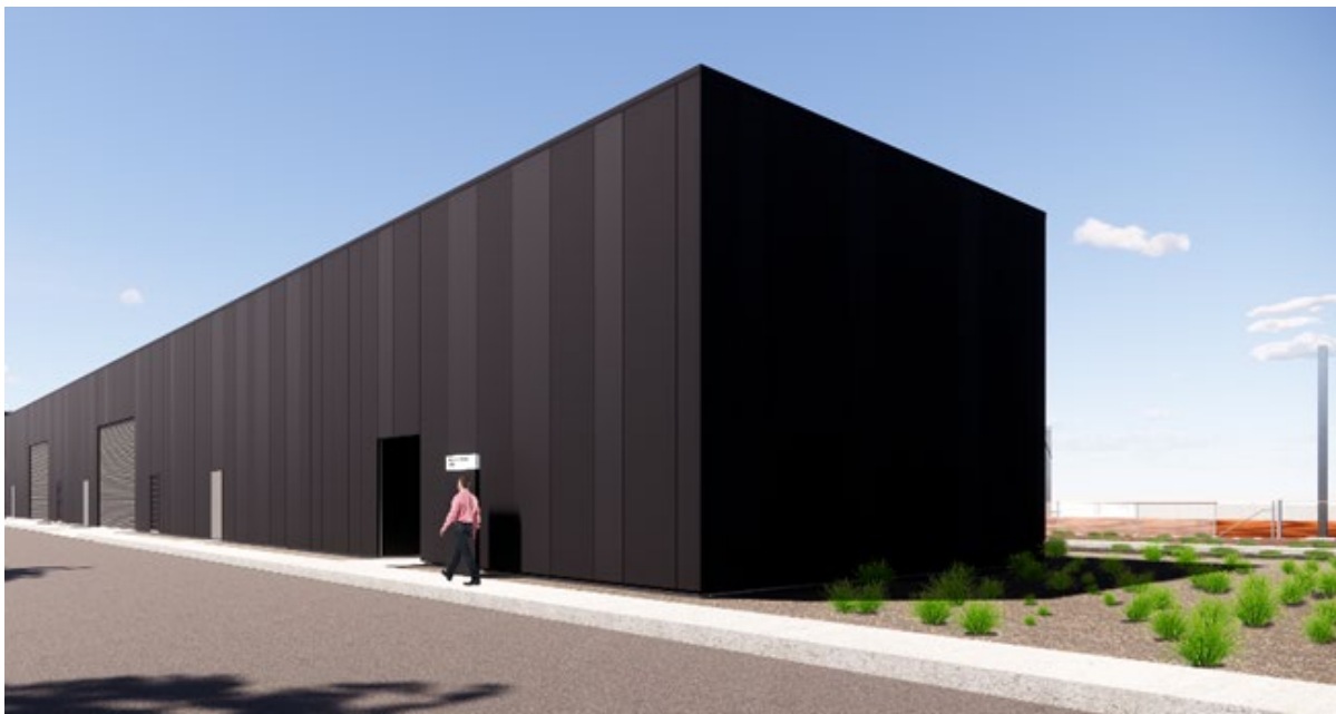
Figure 6-7 SMTFS – Maintenance workshop building viewed from the internal circulation road looking south east
