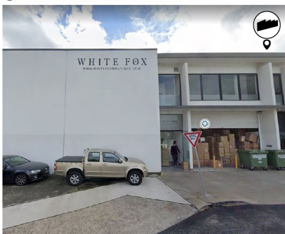
3 215 Edgware Road - Industrial Context
