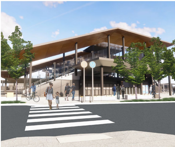
1 Sydenham Station Works
