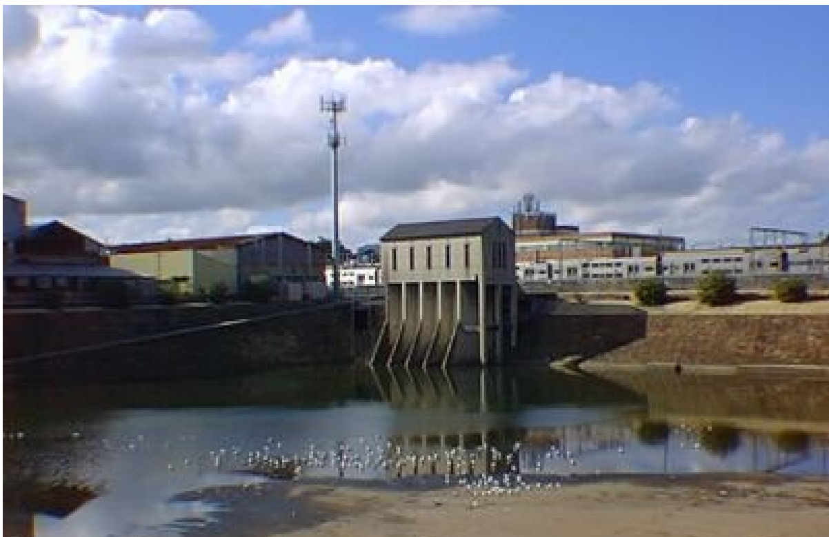
Figure 4-2 Sydenham Pit and Pumping Station – View of pit with pump house in background. Image by James Stephany. Image copyright owner Sydney Water Corporation.
