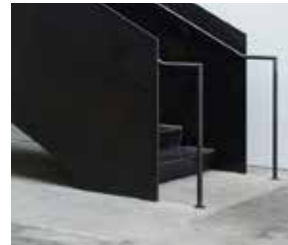
3. Charcoal Steel feature Stair
