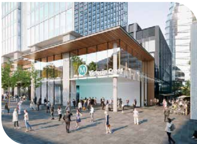
The main Victoria Cross Metro Station entrance from the primary plaza fronting Miller Street. Integrated with the public domain and the new through site link.
