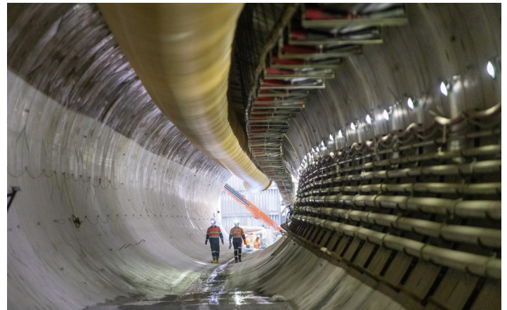
Conveyor structures and service pipes.
