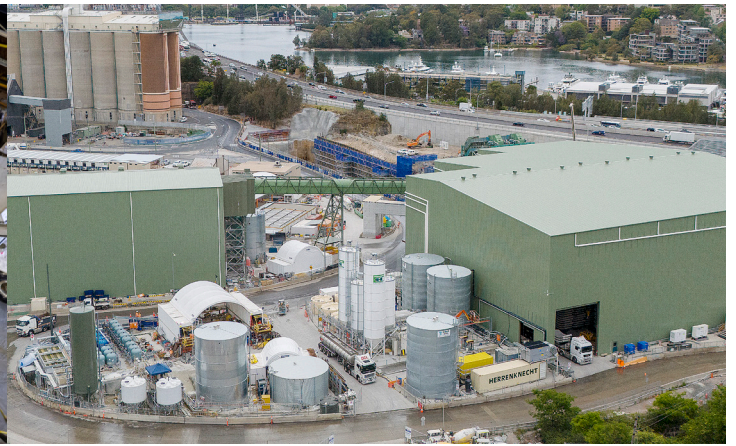
Grout batching plant at The Bays.
