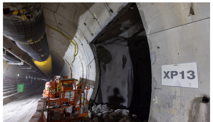
A cross passage connecting the two metro tunnels under Rozelle.
