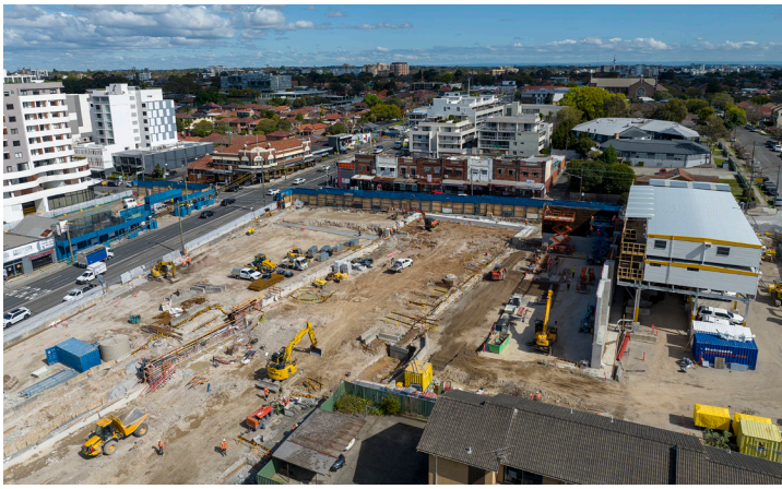
Burwood North site before major excavation started (August 2022).
