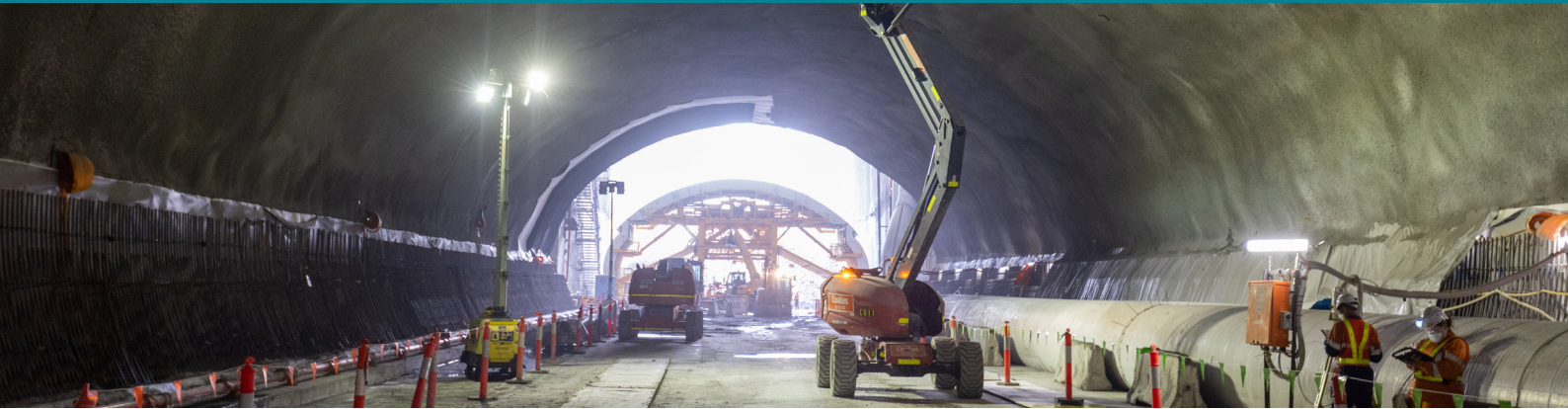
Burwood North crossover cavern.
