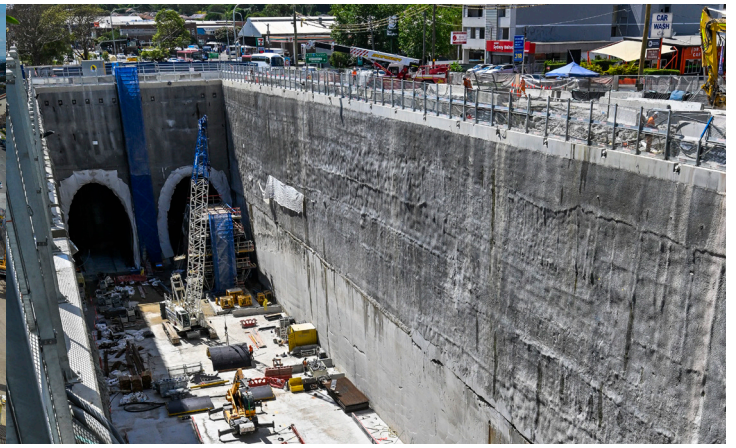
Excavated station box at Burwood North site (December 2023).
