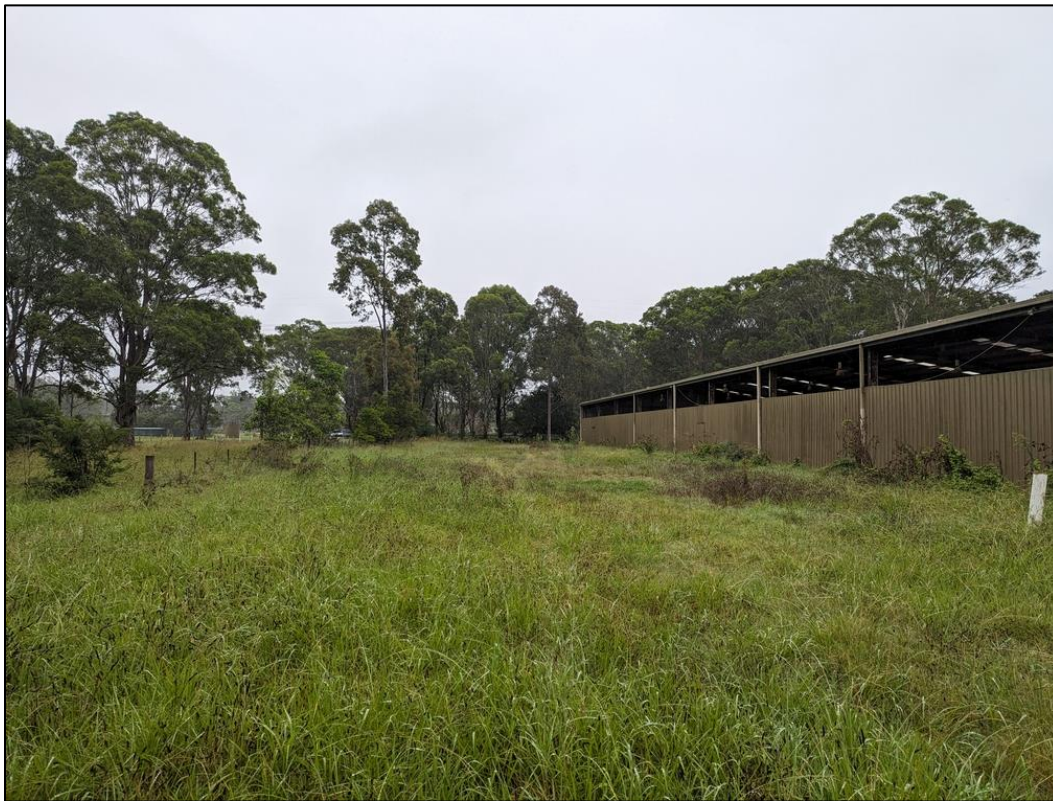
Photograph 1: Showing the property at the end of Samuel Marsden Road where the proposed sewer main will connect to the existing Sydney Water DN1350 submain. The existing farm building is visible on the right of the photo.
