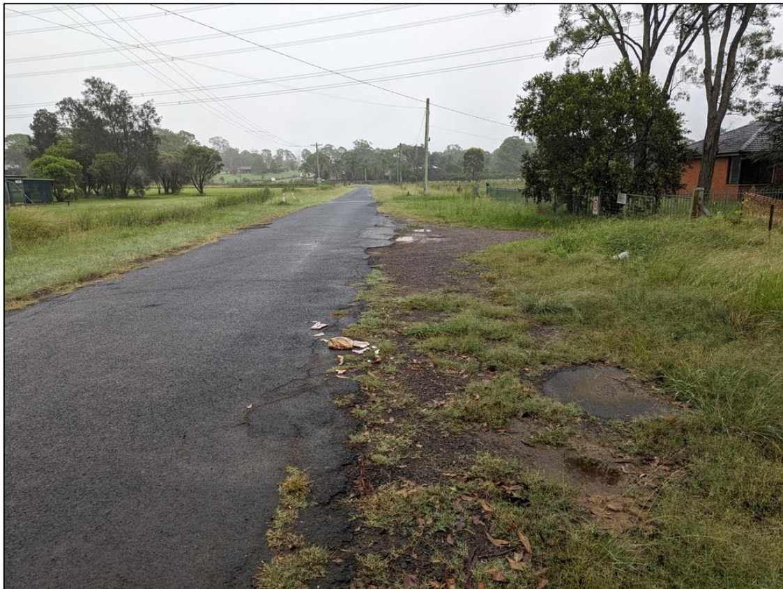
Photograph 6: Facing west and looking along the road reserve of Samuel Marsden Road where the proposed sewer main will be constructed.
