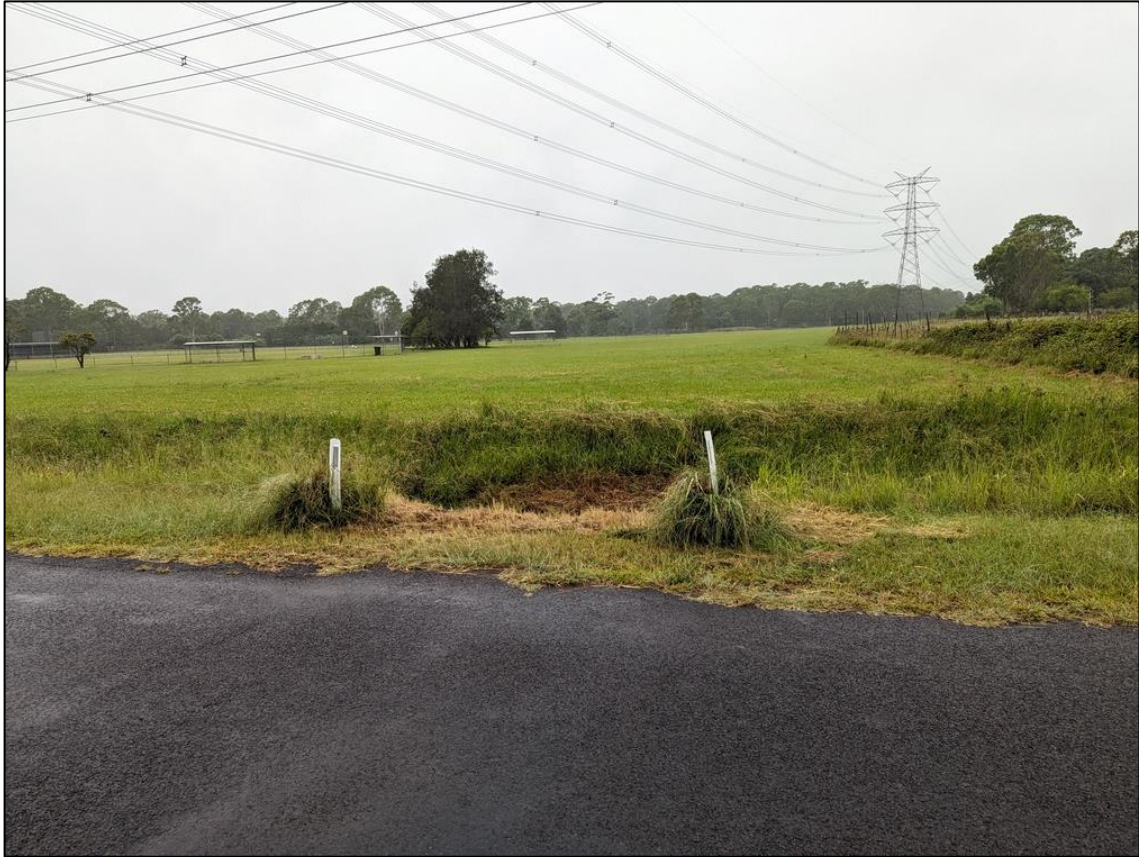
Photograph 7: Showing evidence of drainage channels within the road reserve.
