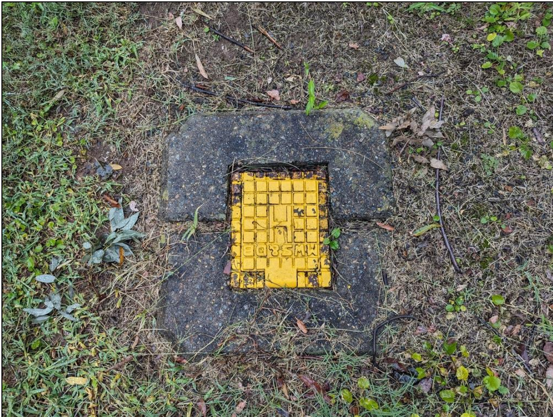
Photograph 10: Showing evidence of underground services within the road reserve of Lansdowne Road.
