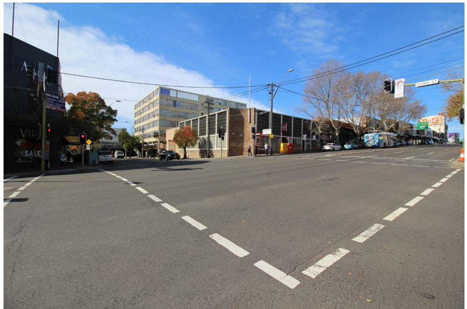
05 Pre-construction view east from corner of the Pacific Highway and Hume Street
